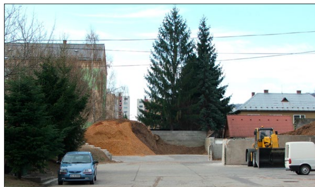
Figure 2: Biomass storage of end user in boiler house.
