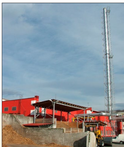
Figure 1: Boiler house in Žarnovica
