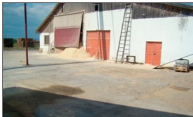
Fig. 3. Facility for wood chips production
